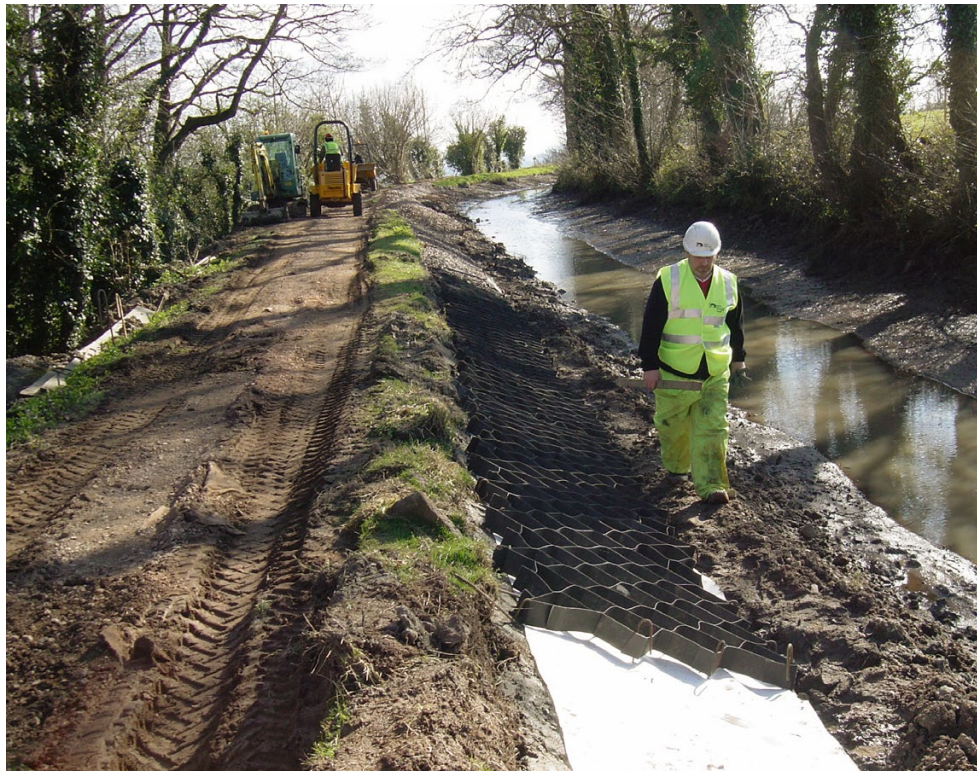
FIGURE 8 TYPAR Geocell CS systems are permeable to water, air and nutrients for better stability and vegetative performance. Photo courtesy TYPAR Geosynthetics.
