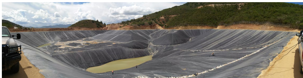
FIGURE 11 Geomembrane liners for heap leach pads cover the Don David goldmine in Oaxaca, Mexico. Photo courtesy of ATARFIL.
