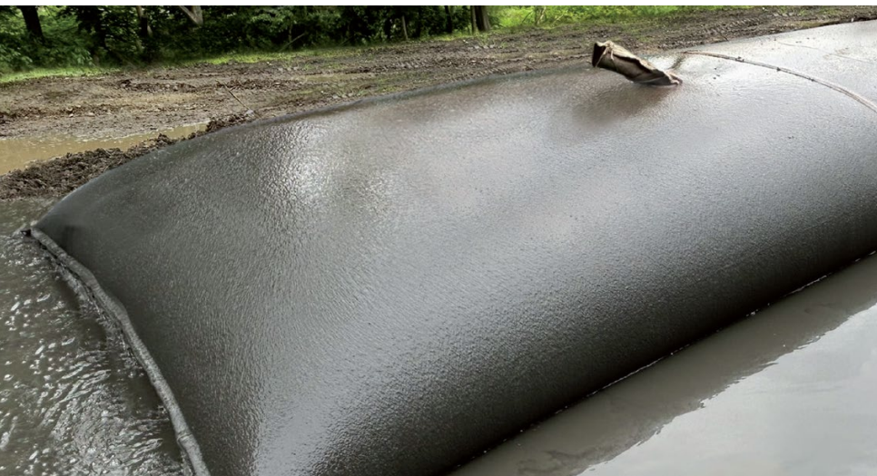
FIGURE 4 Dewatering tubes made from SoilTain offer flexible filling quantity, high absorption capacity per hour, high dry residue, processing without intermediate storage and low use of resources. Photo courtesy of HUESKER.
