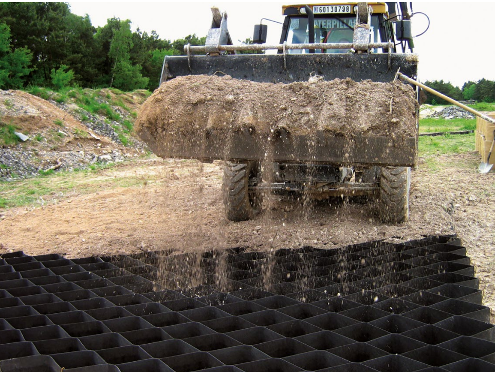
FIGURE 7 TYPAR's geocell ground stabilization systems ship in compacted panel form and expand into honeycomb formations to the desired shape and dimension on-site. Photo courtesy TYPAR Geosynthetics.
