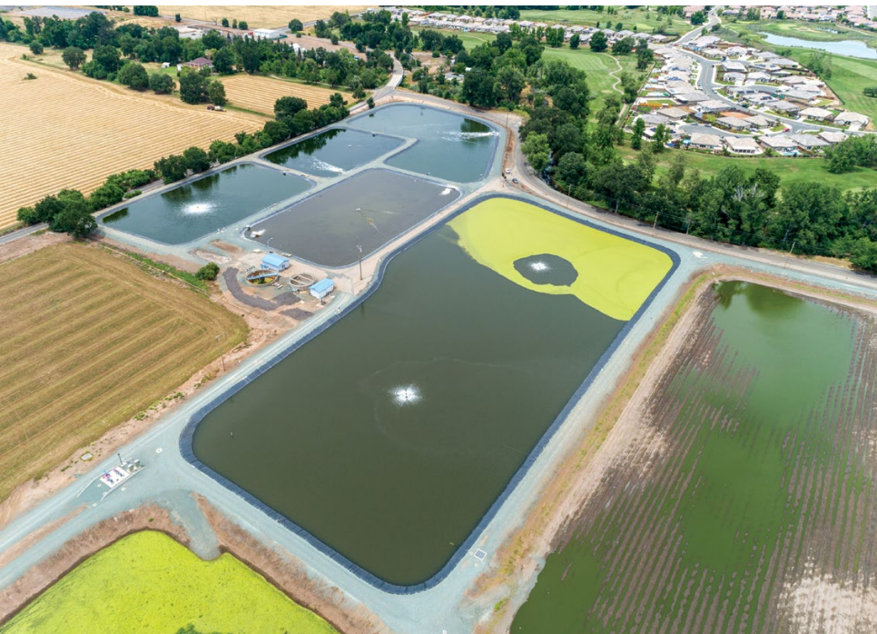
FIGURE 6 Wastewater treatment ponds in Lone, Calif. Photo courtesy of Viaflex.
