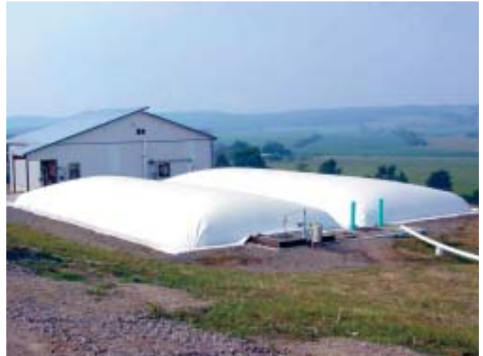
Photo 1. Animal waste lagoons produce toxic emissions (e.g., ammonia and hydrogen sulfide). Geosynthetic cover systems can contain emissions, and in conjunction with methane conversion equipment produce power for heating structures—barns, houses—and water. Excess power can be sold to local grids.
