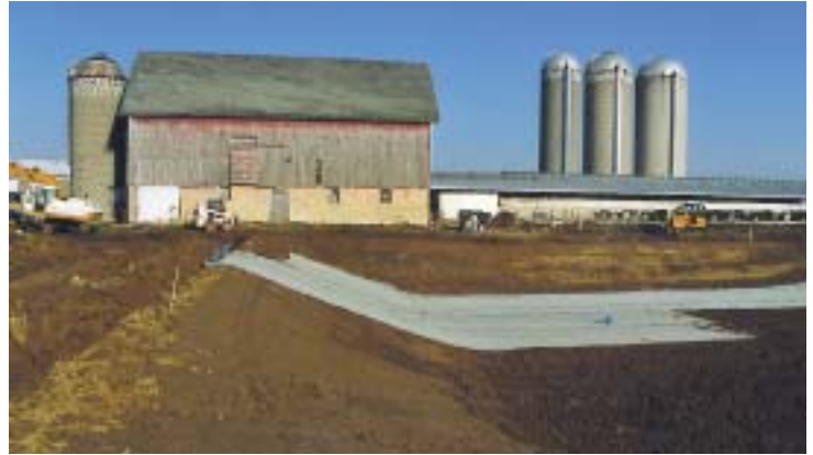
Photo 2. Geosynthetic clay liner was installed at this farm in Minnesota.
