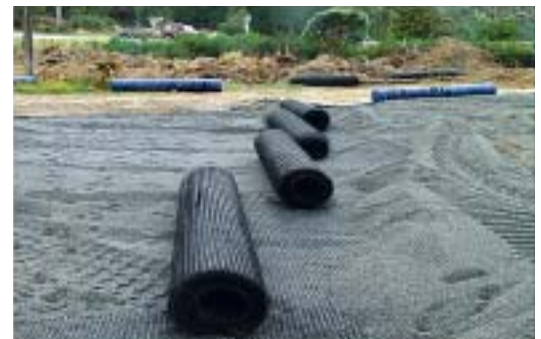
Photo 1. Placement of geogrids.
