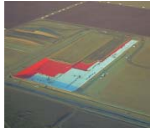
Photo 1. Aerial photo of Visalia WMU-2 under construction.
