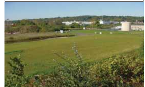
Photo 6. Completed final cover.
