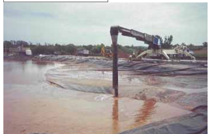
Photo 4. Placement of soil.
