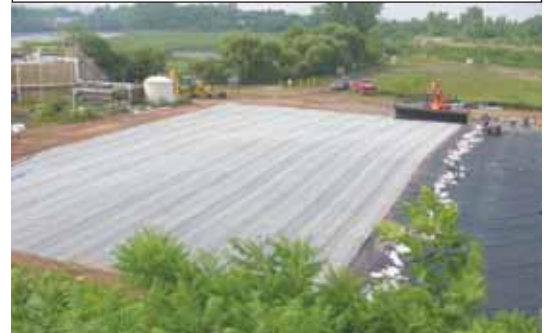
Photo 5. Geomembrane installation.
