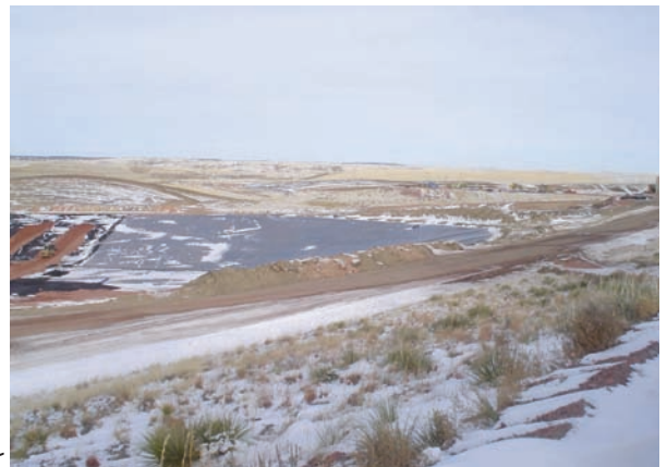
Photo 4. The installer's experience helped complete the project on time and under budget.
